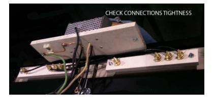
Inspect the terminal enclosure and conduit connections for evidence of water leaks or moisture collection. Tighten connections as required. Clean up any corrosion. Do not continue using a heater with signs of damage.
